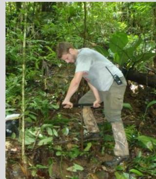
Figure 3: Drilling borehole for piezometer
